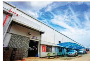
Project Name: STP for Debonair Padding & Quilting Solution Ltd (DPQSL) Capacity: 70 m 3 /day Location: New DOHS, Mohakhali
