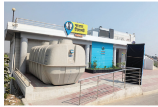
Project Name: Potenga Sea Beach Public Toilet Capacity: 15 m 3 /day Location: Patenga Sea Beach, Chattogram
