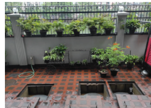
Project Name: Saif Mansion (ABC House) Capacity: 5 m 3 /day Location: Gulshan 02
