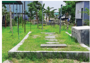
Project Name: 6-Brigade Capacity: 40 m 3 /day
