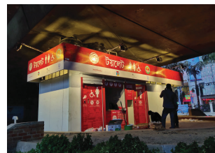
Project Name: Mohakhali Public Toilet Capacity: 5m 3 /day Location: Mohakhali Rail Crossing
