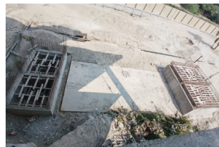
Project Name: STP for Rangpur Novotheater Capacity: 150 m 3 /day Location: Rangpur
