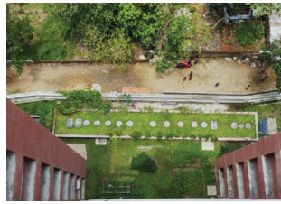
Project Name: Cox's Bazar Development Authority Capacity: 80 m 3 /day Location: Cox's Bazar
