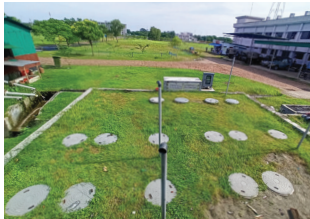
Project Name: 7 FI (Lady Barrack) Capacity: 40 m 3 /day
