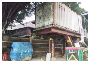
Project Name: Smart Traffic Police box (Mirpur-13) Capacity: 2 m 3 /day Location: DNCC
