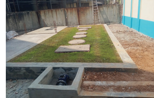
Project Name: Bay Footware Capacity: 30 m 3 /day Location: Mouchak, Kaliakair, Gazipur-1700
