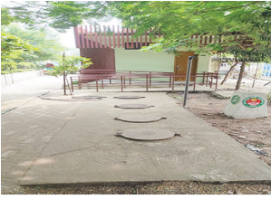
Project Name: Lawtola Khal Public Toilet Capacity: 2 m 3 /day Location: Bosila Mohammadpur
