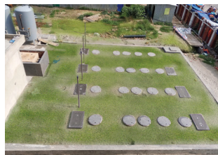
Project Name: Paikpara Govt. Officers Building Capacity: 1050 m 3 /day Location: Paikpara, Mirpur 1
