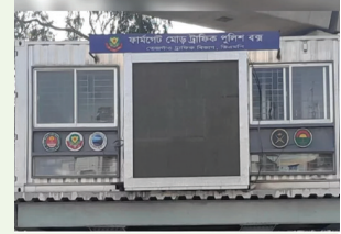
Project Name: Smart Police Box. Type : Container type police box. Units : 4 Nos. Location : Agargaon, Asadgate, Shyamoli, Gulshan 1
