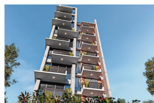
Project Name: STP for Fatematuzzohra Residence Capacity: 5 m 3 /day Location: Bashundhara Residential Area
