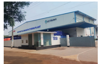
Project Name: STP for Yamaha Manufacturing Plant Capacity: 50 m 3 /day Location: Rajendropur, Gazipur
